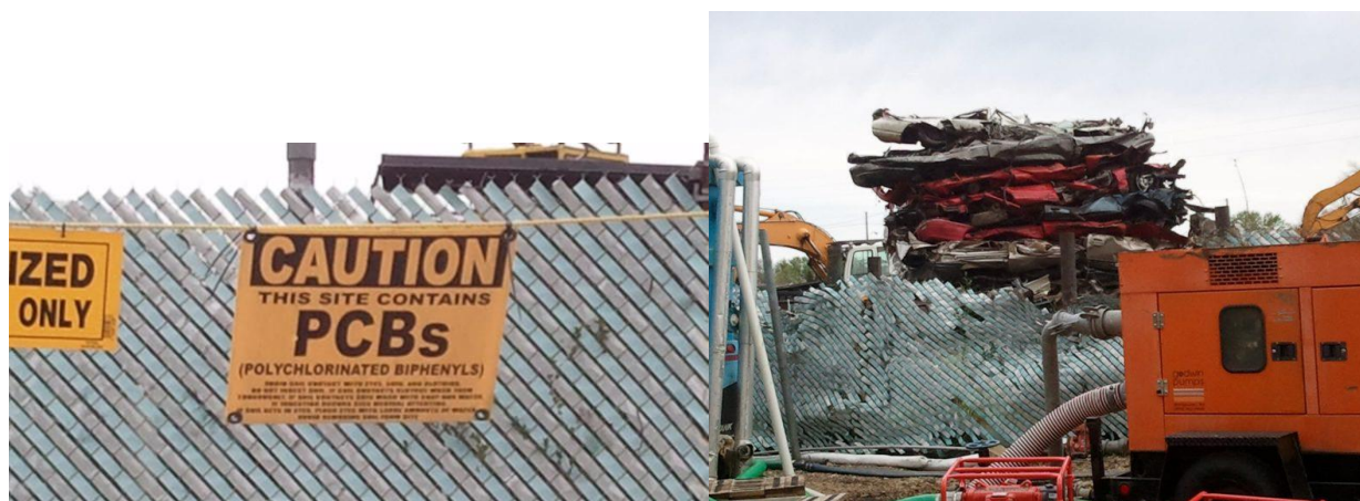
A sign at the Hartford Iron & Metal plant warning of PCBs, or polychlorinated biphenyls.
